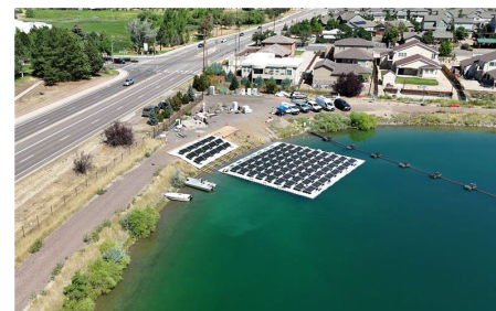
50kW pilot of tracker to increase energy production by >10%
